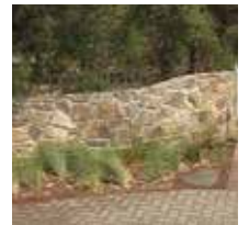
Once clean, re-apply WBGC.
