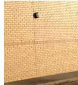
Mural removal after spraying TRANSGEL with airless paint sprayer.
