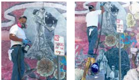
MURALSHIELD being applied with HVLP sprayer
